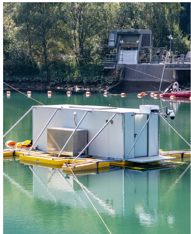
Sediment is dredged via the dredging platform and discharged systematically to the Drau river.
