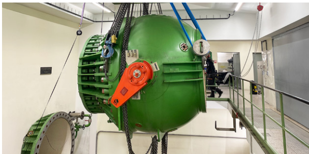
Removal of the spherical valve at the Imst power station.
