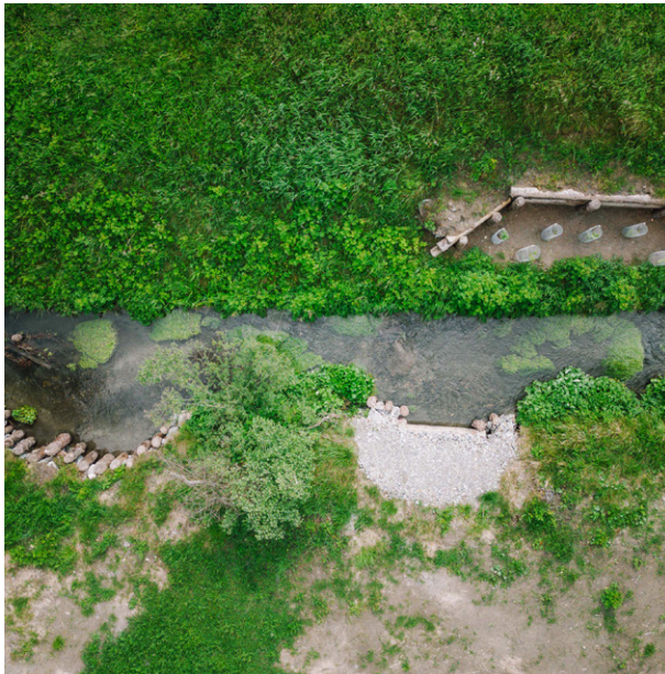
Structuring measures on the Bürgerau drainage ditch near Matriei
