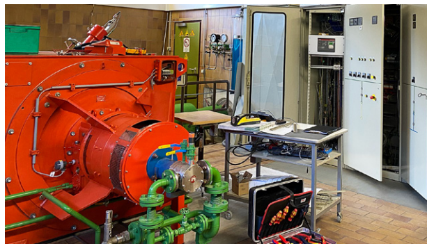
The generator at the Urgbach power station was cleaned using dry ice, among other methods.
