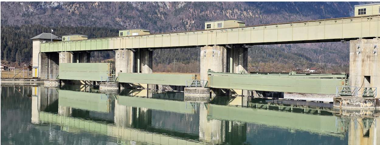
The stop logs at the Kirchbichl weir were still made of wooden planks.
