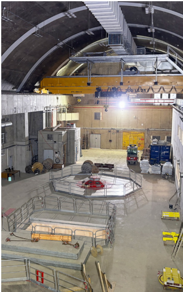
Concrete work in the cavern was completed.
