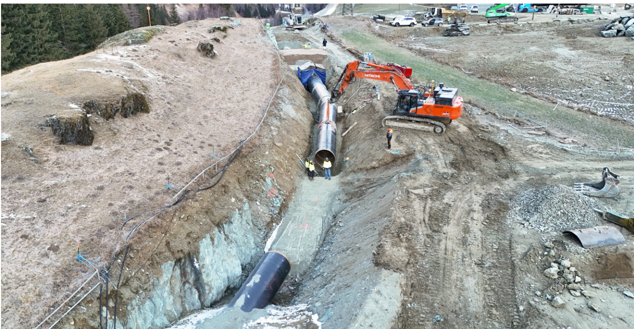
Installation of the last pipe of the penstock in December 2025
