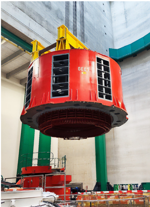
The old stator is being removed ...
