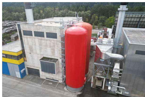
The buffer tank at the Lienz biomass heating plant is being expanded.
