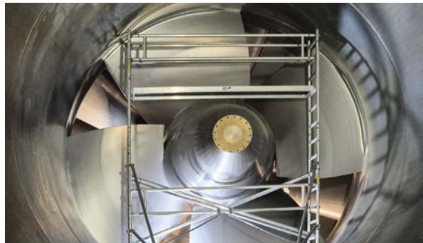
Also the runner blades were inspected as part of the overhaul at the Langkampfen power station.
