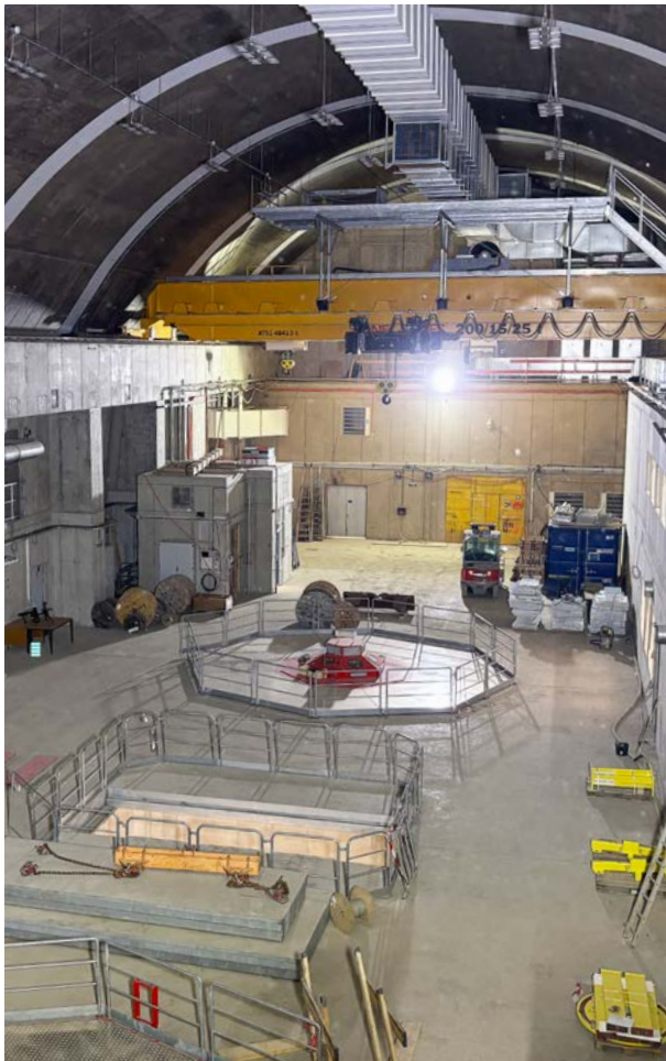
Concrete work in the cavern was completed.
