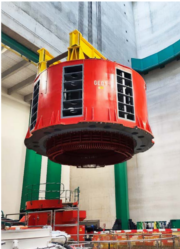
The old stator is being removed ...
