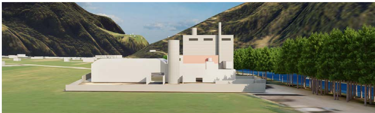
The new Längenfeld heating plant
