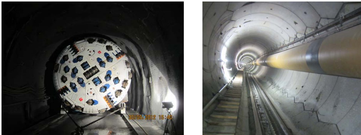
Figure 3: TBM-DS (l.) and segmental lined shaft (r.)
