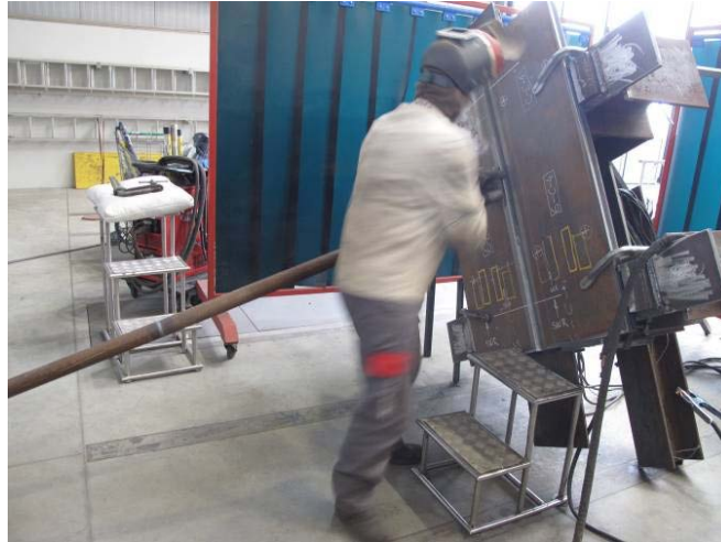
Figure 3: Welding of plain plates in upwards position and 30° inclination
