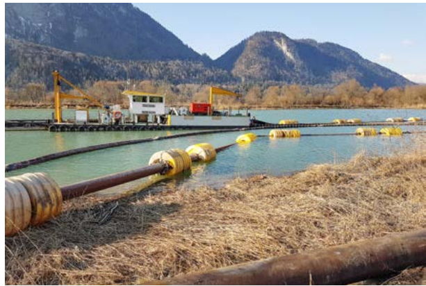
Dredger at Langkampfen power station
