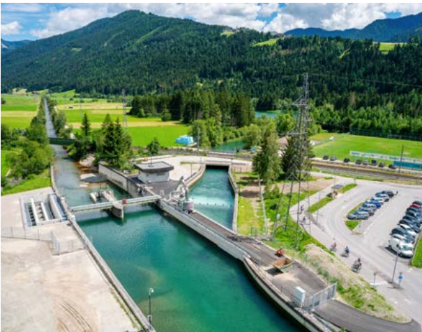
The generally overhauled Tassenbach weir
