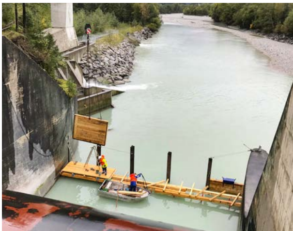
Sealing of the weir against tailwater
