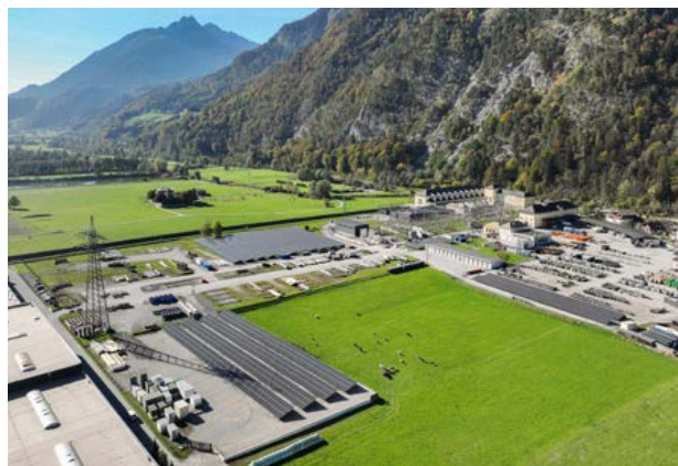
At a capacity of 1.7 MWp, the solar power station in Jenbach is one of the biggest PV stations in Western Austria.
