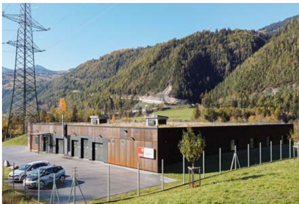
The GKI power house in Prutz upon completion.
