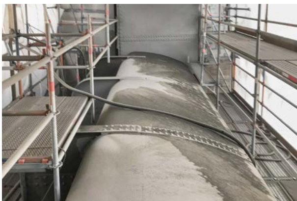
Scaffolding and housing
