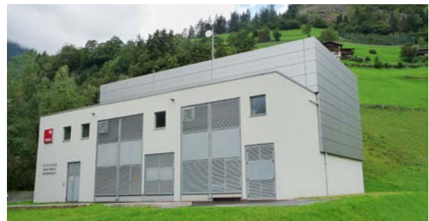
The power house of Schwarzach power station in Huben, East Tyrol upon completion
