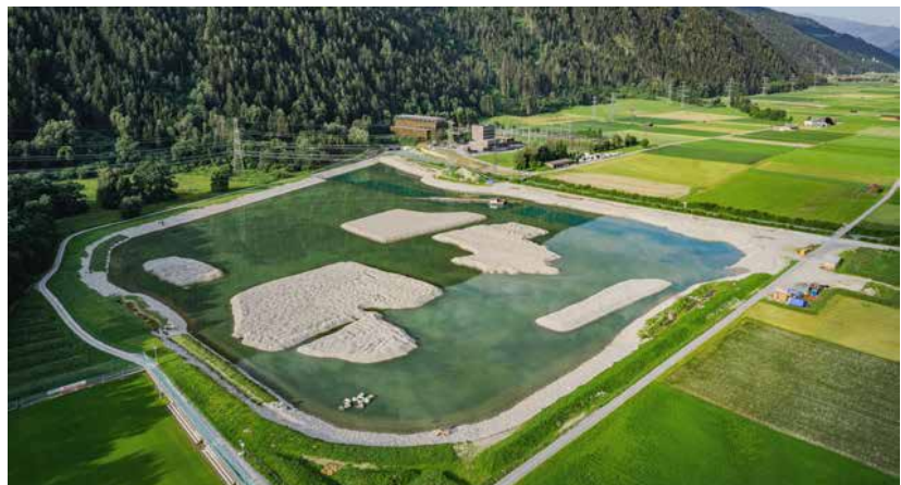
The tailwater reservoir under construction at the Silz power station
