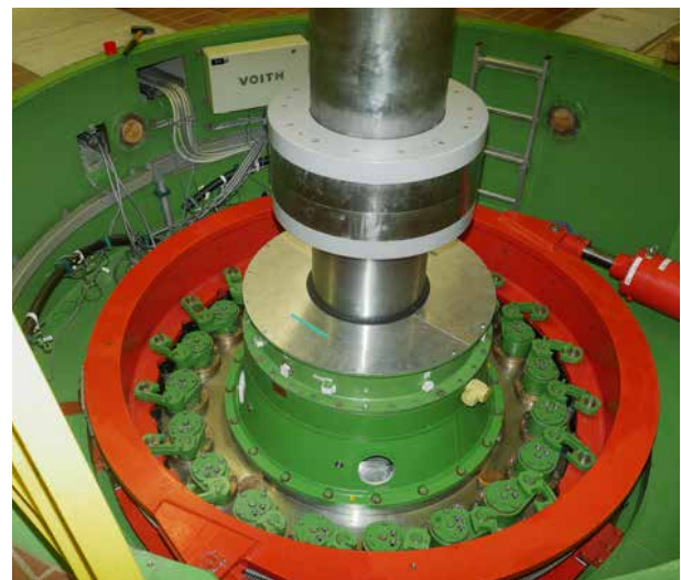
The compact part of the turbine was lifted out, completely refurbished, and reassembled.
