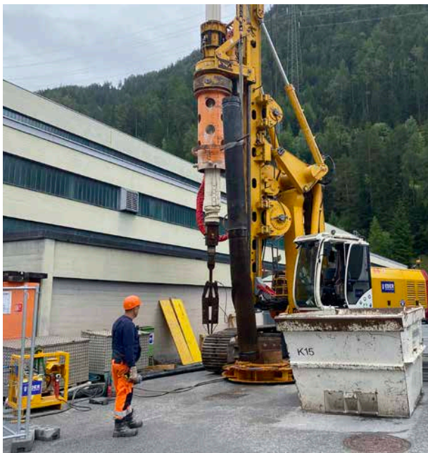
Old filter pipes were removed and replaced by new stainless steel ones.
